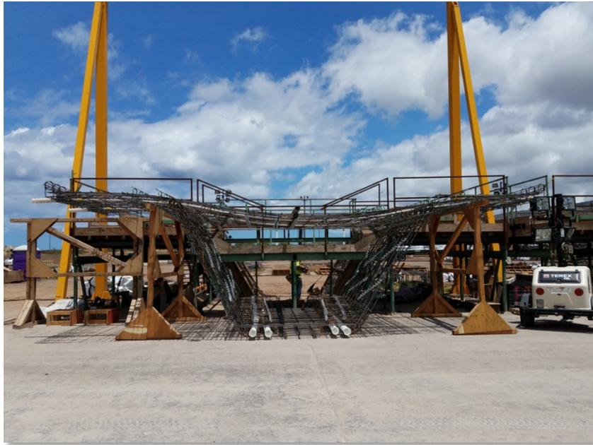
*Note SDI's Corrugated PT Duct (white) running both longitudinally and horizontally in this form for a precast segment of the train's elevated guideway.*
