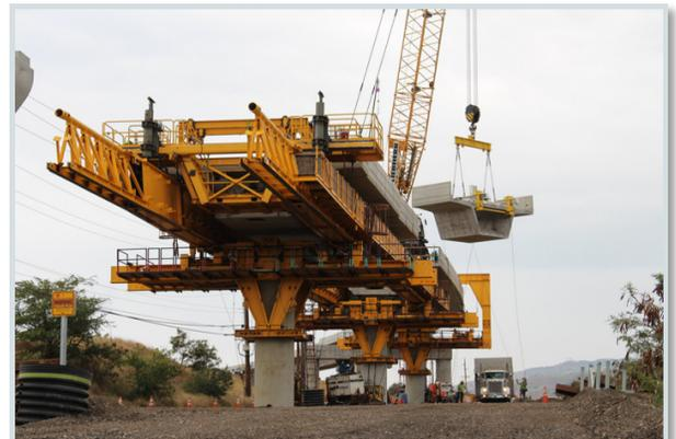
*Precast segment of the elevated guideway being lifted into place. Post-tensioning will then be applied.*
