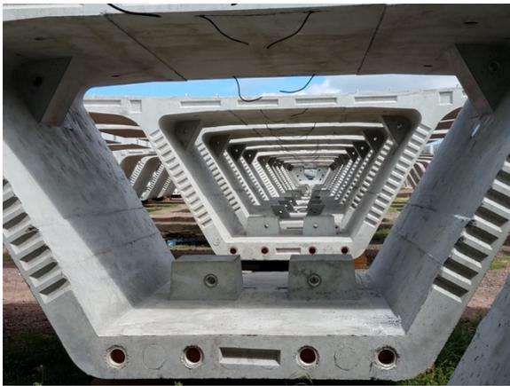
*SDI's duct is visible here, and soon these precast segments will be lifted and tensioned together with post-tensioning strand (also supplied by SDI).*
