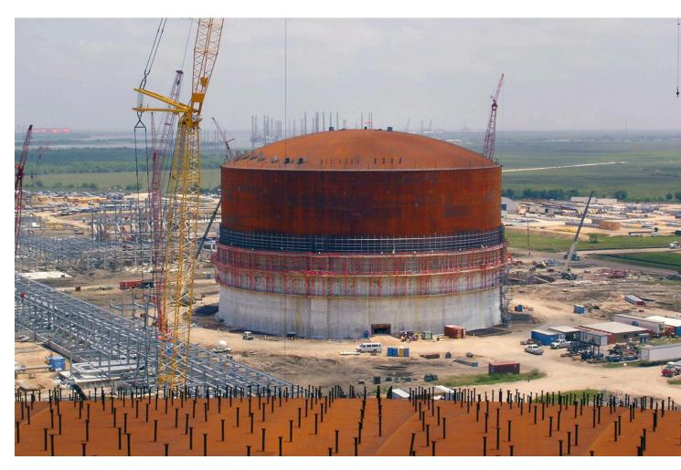
SDI'S POST-TENSIONING WORK FOR THE GOLDEN PASS LNG TERMINAL PROJECT WAS SUCCESSFULLY EXECUTED WHILE WORKING UNDER AN EXTREMELY DEMANDING FAST-TRACK SCHEDULE AND THE NEED TO DESIGN AND PERFORM A COMPREHENSIVE CRYOGENIC TESTING PROGRAM TO QUALIFY THE POST-TENSIONING SYSTEM. SDI ALSO PERFORMED SITE CLEANUP AND RECOVERY WORK AFTER A CATEGORY 4 HURRICANE DEVASTATED THE AREA WITH STORM SURGES AND HIGH WINDS.
