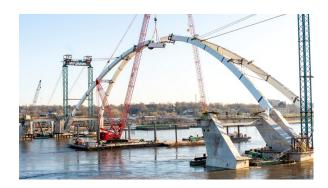
To facilitate temporary stay installation, SDI engineers specially designed threaded anchor ring nuts, post blocking devices, cable clamps, and performed proof load testing. The SDI shop then made necessary adjustments to the installation equipment (modifications, calibrations, setup) to suit the specially designed hardware.
