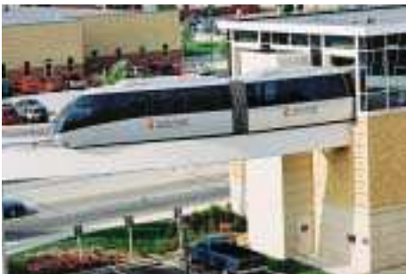
The Methodist Hospital Station, northern most on the APM route, features a passenger platform and safety and security Control Center on its upper level. The system's maintenance facility is on the lower level, as is power distribution equipment and the People Mover's back-up generator.
