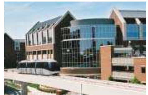
The southern most, IU/Riley Station serves the University Medical Center, Riley Hospital for Children, and the entire campus area. Because adjacent projects were already underway, SDI coordinated its construction schedule with all involved parties through bi-weekly meetings.
