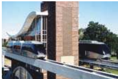
The Canal Station on 11th Street will eventually serve facilities in a planned life sciences complex, including a biotech research facility and a 180,000 sq. ft. Clarian medical lab. To accommodate connection with anticipated structures, SDI incorporated future walkway provisions into the station design.
