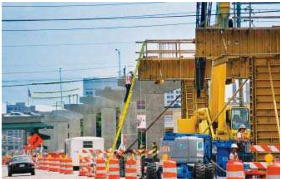
The total scope of work under SDI's design/build contract included all traffic control and traffic control devices required to minimize negative impacts of construction on the city's established traffic-flow patterns.
